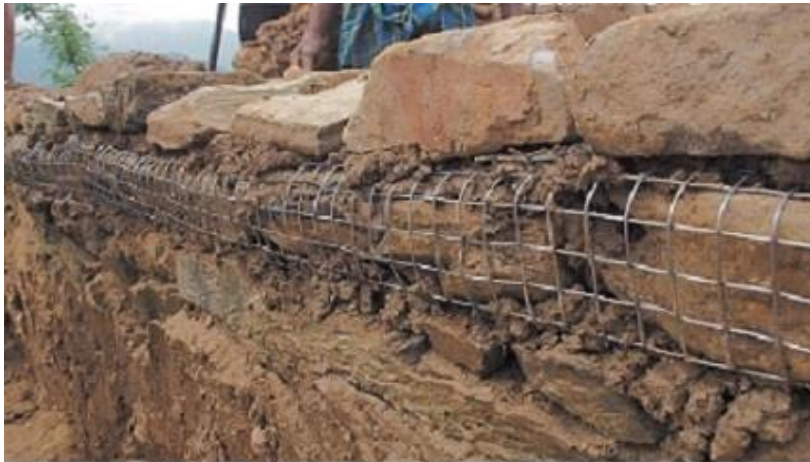
Gabion Band wrapped with wire
