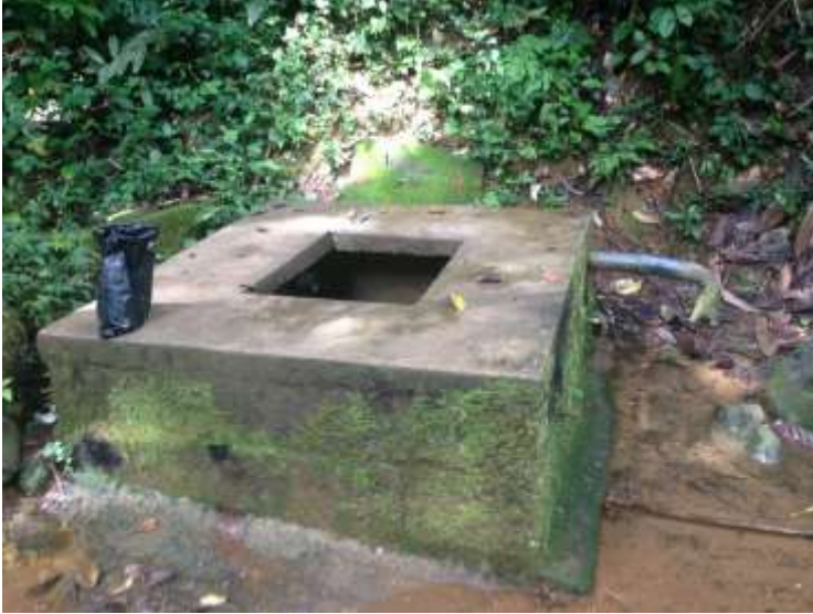
Figure 7. The Monien Ebhe Spring does not have a single owner, it is property of the whole village. It has a concrete catchment. At time of testing, no E. Coli was found at the source, only in the spring water stored in houses.
