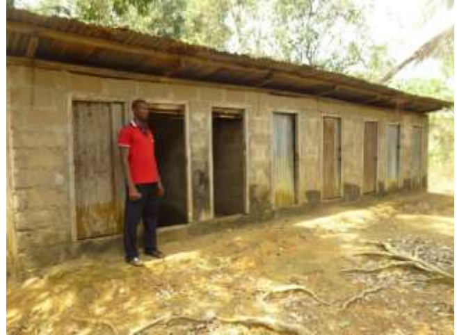
Figure 18. Group of latrines for a large compound serving multiple units.
