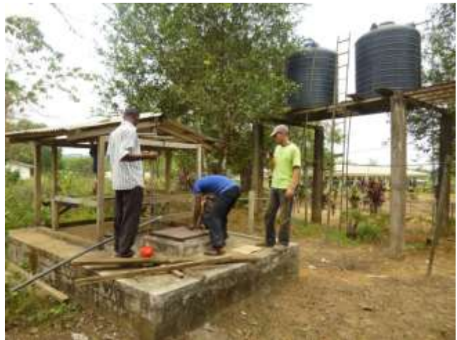
Figure 12. Rogerio, Takor and Clinic Groundskeeper examining the spring catchment at the Presbyterian Health Clinic. The water is pumped up to the storage tanks
