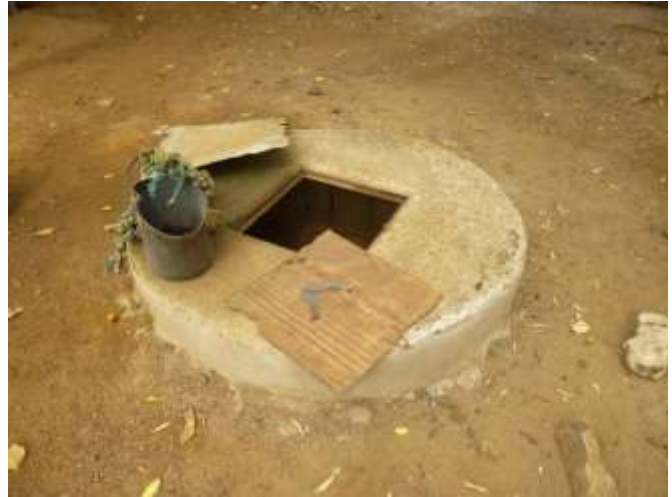
Figure 4. Typical well showing concrete skirt around the well and cover.
